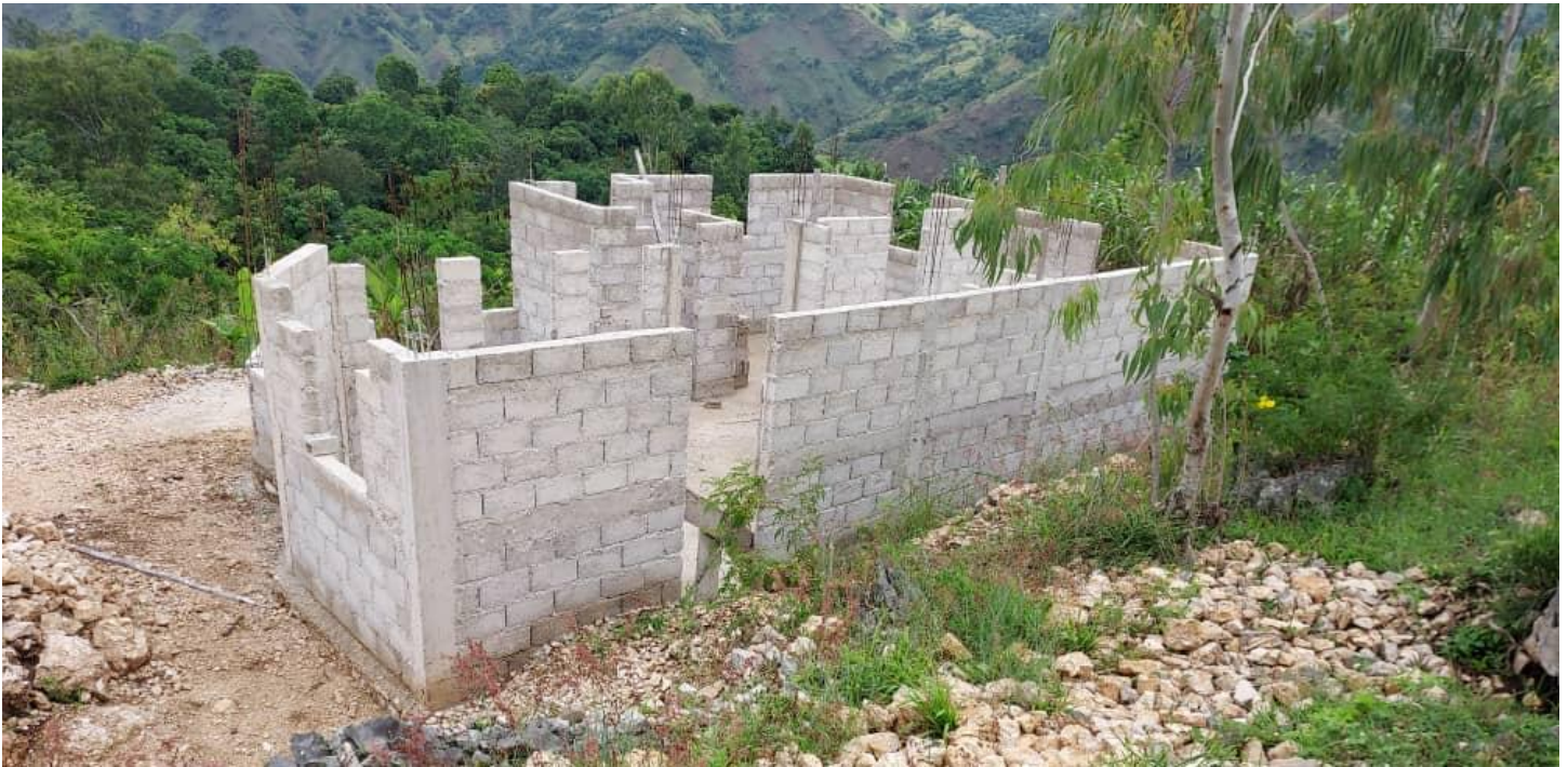
Jonique's House under construction.
