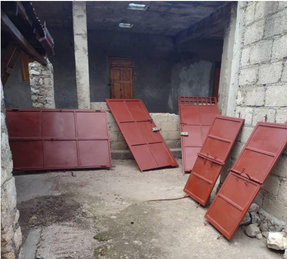
Immaculate Conception - Preschool Construction - Doors and windows ready.
